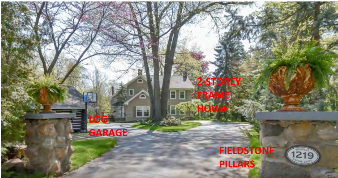
Entrance from Ravine Drive
